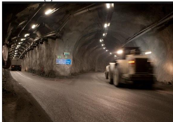
Figure 1. LEDs arrays in underground mine
