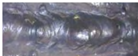
Figure 10. An example of welding defects classified as excessive reinforcement.
