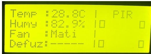
Figure 10. Off Fan Condition
